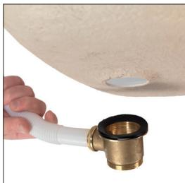
3. Offer the bath waste into position ensuring the rubber washer is correctly aligned between the waste assembly and the bath base.
