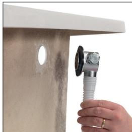
5. Offer the outlet body assembly into position at the rear of the bath ensuring the rubber washer is correctly aligned between the outlet body assembly and bath wall.
