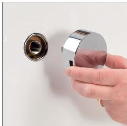
6. Ensuring the rubber washer is correctly aligned, pass the overflow filler outlet through the bath and secure to the body assembly.
