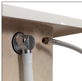
7. Remove the relevant inlet blanking plug and attach the flexible hose to the blended inlet connection.
