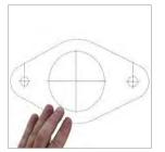
Remove the mounting ring from the rear of the valve using the 2.5mm hexagonal key provided. Locate the ring inside the pre marked position, ensuring the locking screw is in the 6 o'clock position and mark the four fixing holes.
