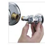
Remove the compression nuts and olives and carefully slide the cover plates onto the elbows. Replace the nuts and olives.
