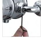
Tighten the inlet compression unions sufficiently to ensure a watertight seal. Push the cover plates over the unions flush to the wall surface.
