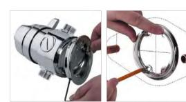
Using a rotary type cutter cut the inlet pipes to length and drill and prepare the fixings for the mounting ring. Fix the mounting ring to the wall using the screws provided.
