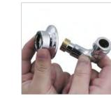
Carefully locate the elbows into the valve inlet connections and push fully home.
